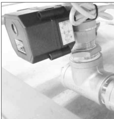
Fig. 6B - Electric Drain Valve
